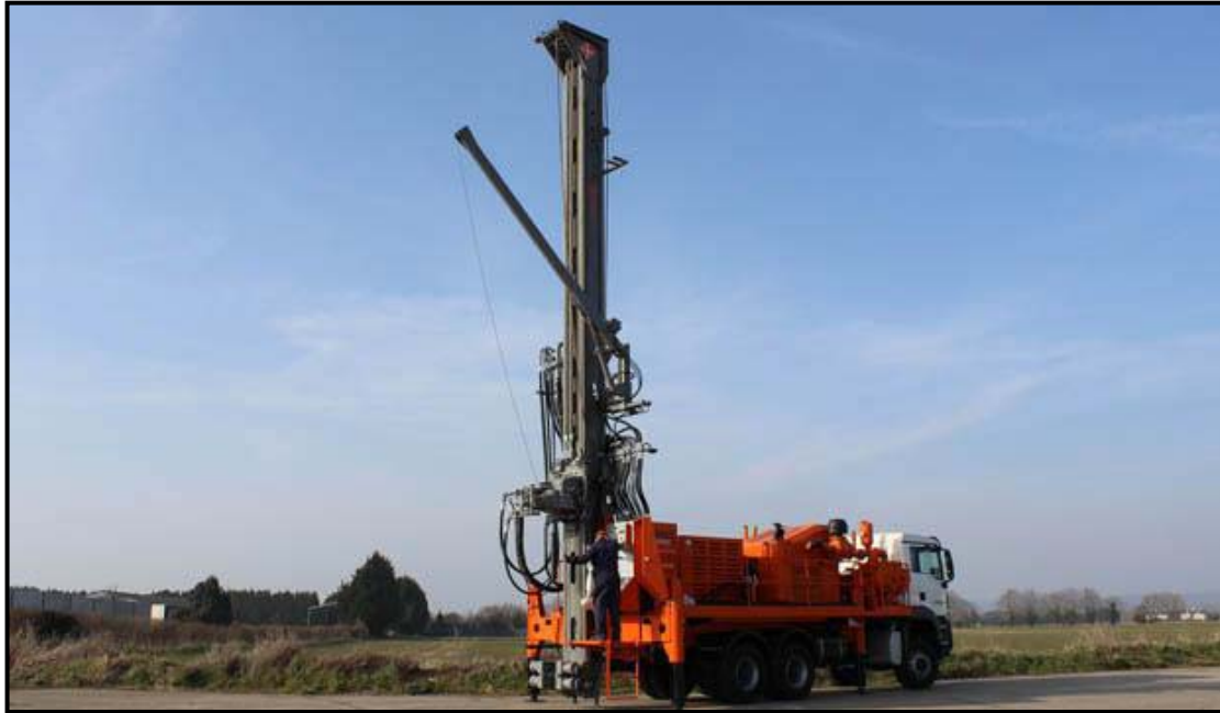
Figure 4 - Photograph of rig vehicle
